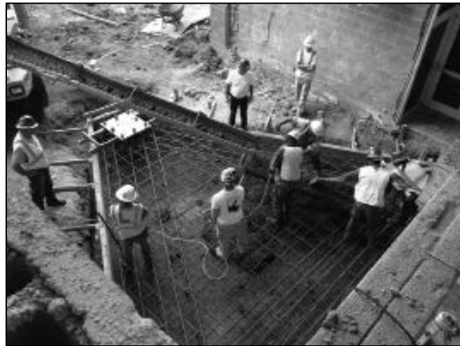
Crews pour telescope pier foundation for State Museum observatory
