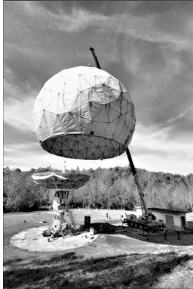
PARI Radome removal from 12-m.
